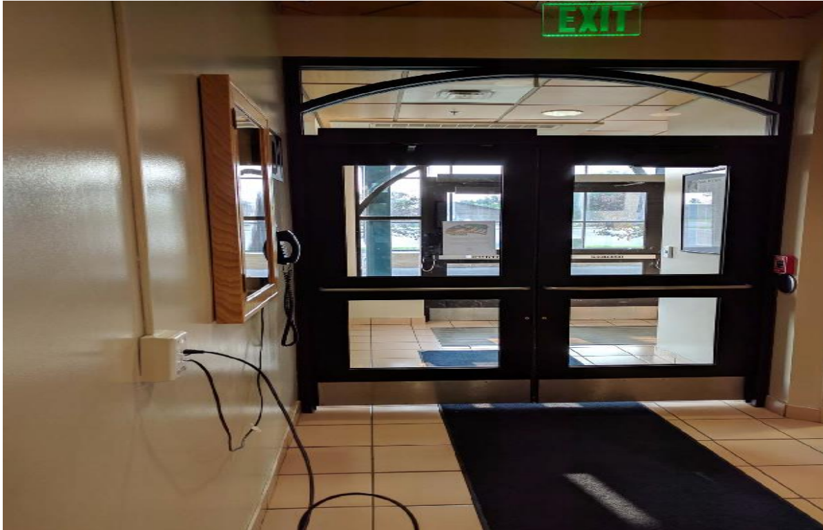
Figure 7: Live network ports in an open area at a hospital that could be used to access the hospital's computer network.
