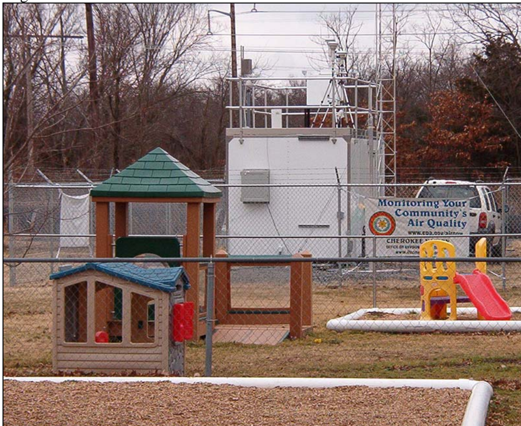
Community Air Monitoring Station
